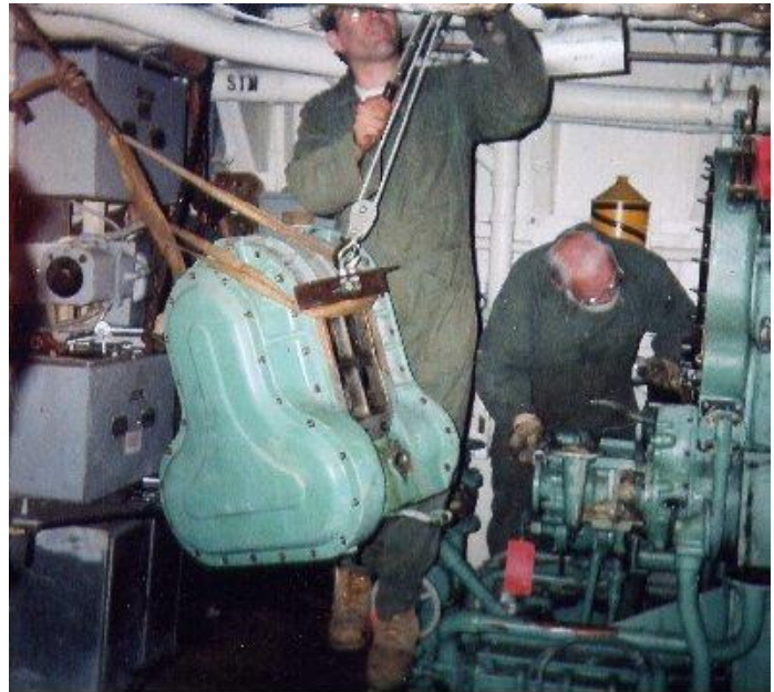
Tearing down the front end of the emergency diesel on the KITTIWAKE.
