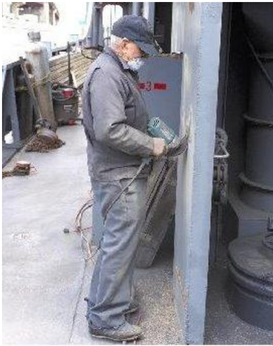
Working towards an autobody finish.
