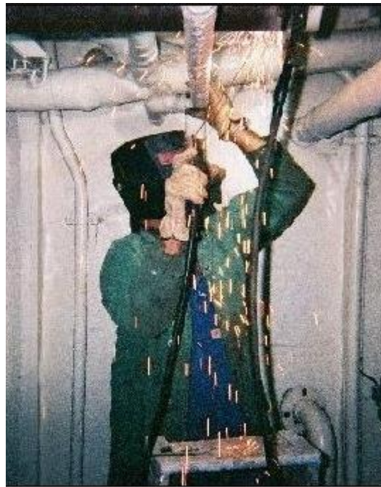
Tom Schriener welding on the sewer discharge line.
