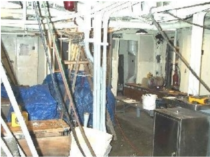
Restoration has started and the messdecks is a mess.
