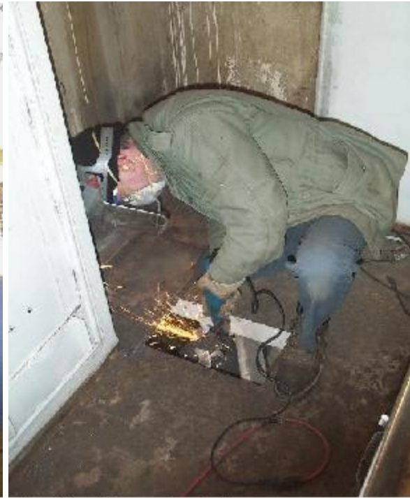
Repairing the pantry deck
