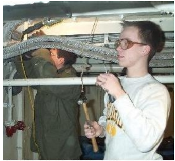
Replacing electrical cable on the messdecks.
