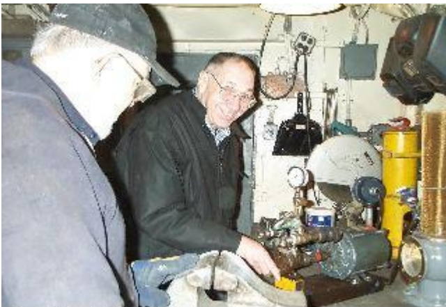
Repairing the fuel oil pump.
