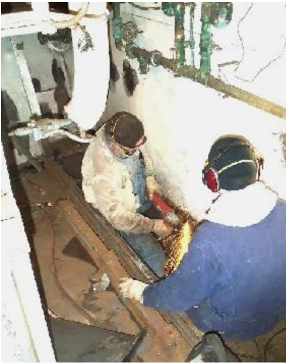
Repairing the reefer deck.
