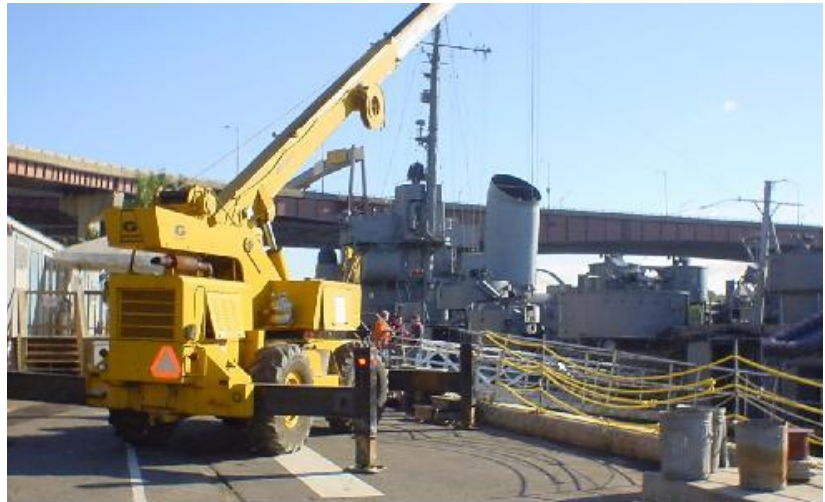
Hoisting the new gangway into position.
