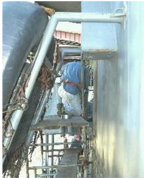
Painting the superstructure.
