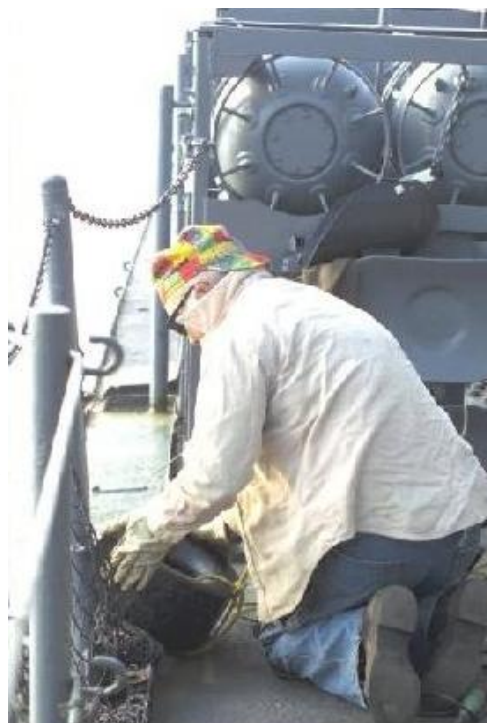
Tanner repairing another chock.
