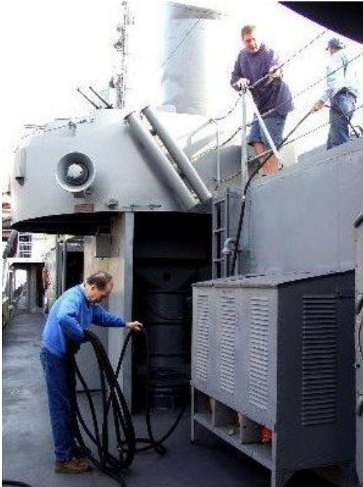
Rigging the washdown hose.
