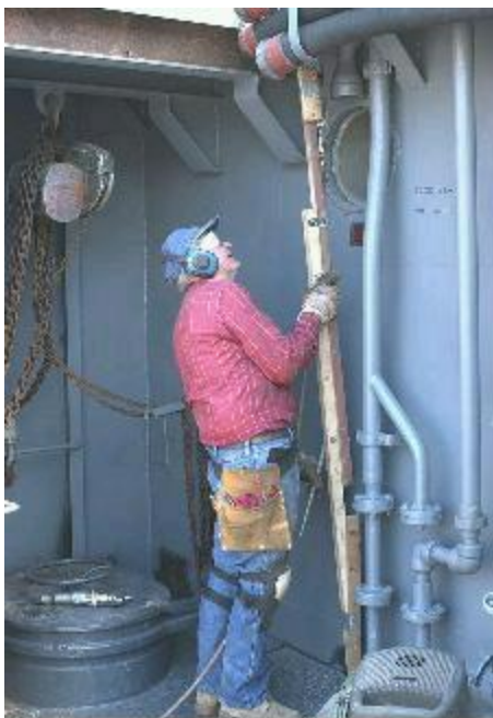
Dick Smith chipping overheads.
