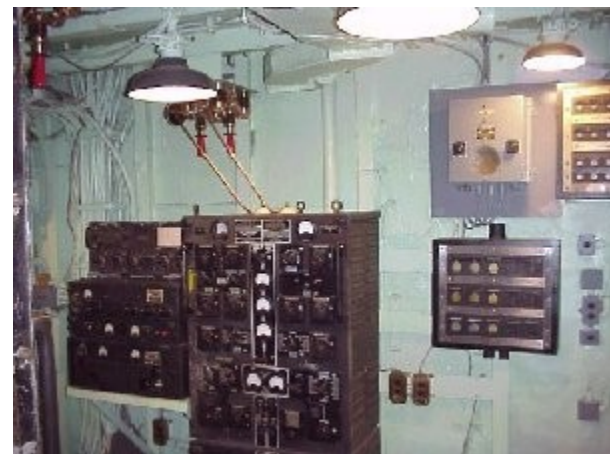
Radio Central - February Restoration Progress
