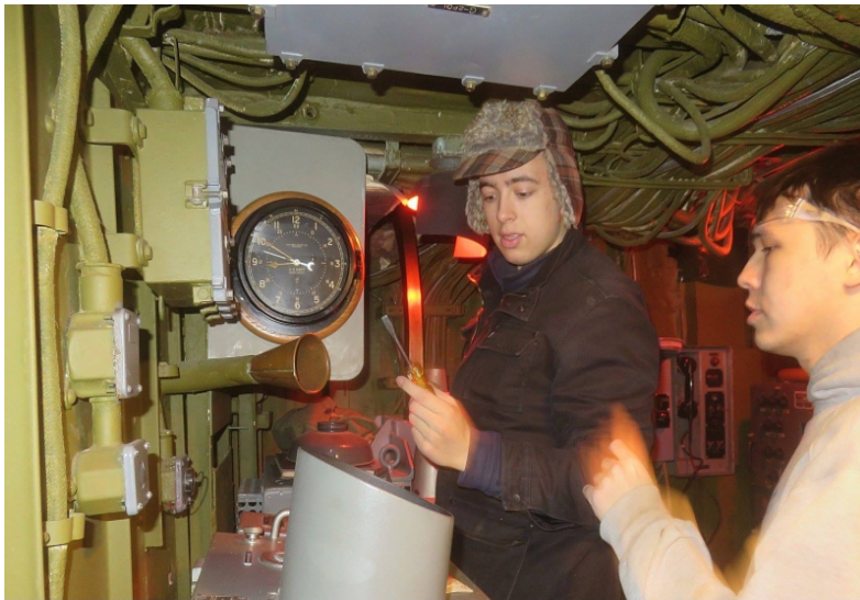
Under Barry Witte's direction, there has been a lot of rewiring in CIC.
