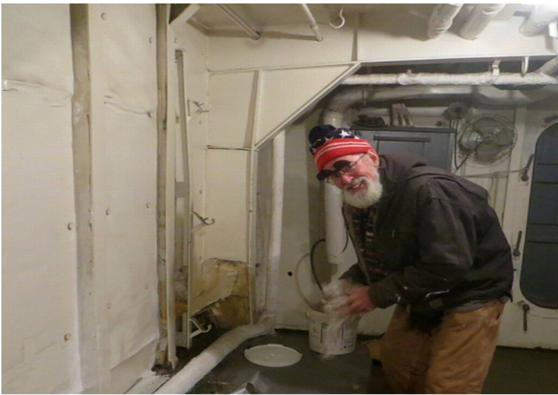
Tommy Moore made repairs to the insulation in the berthing compartment.
