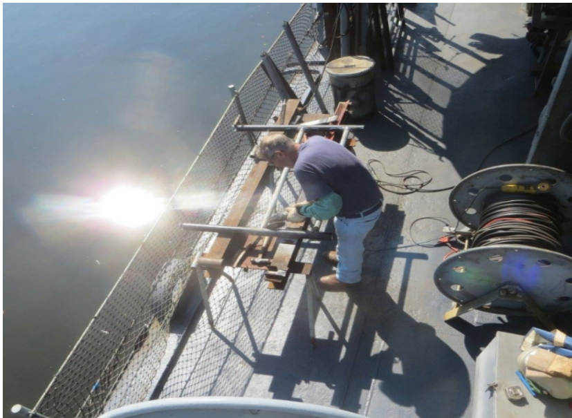
Danny Statile fabricates another section of safety rail for the seawall.
