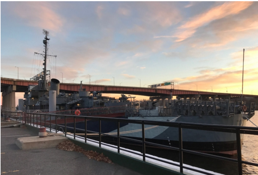
The new seawall safety rail was a big accomplishment of the 2017 Season.
