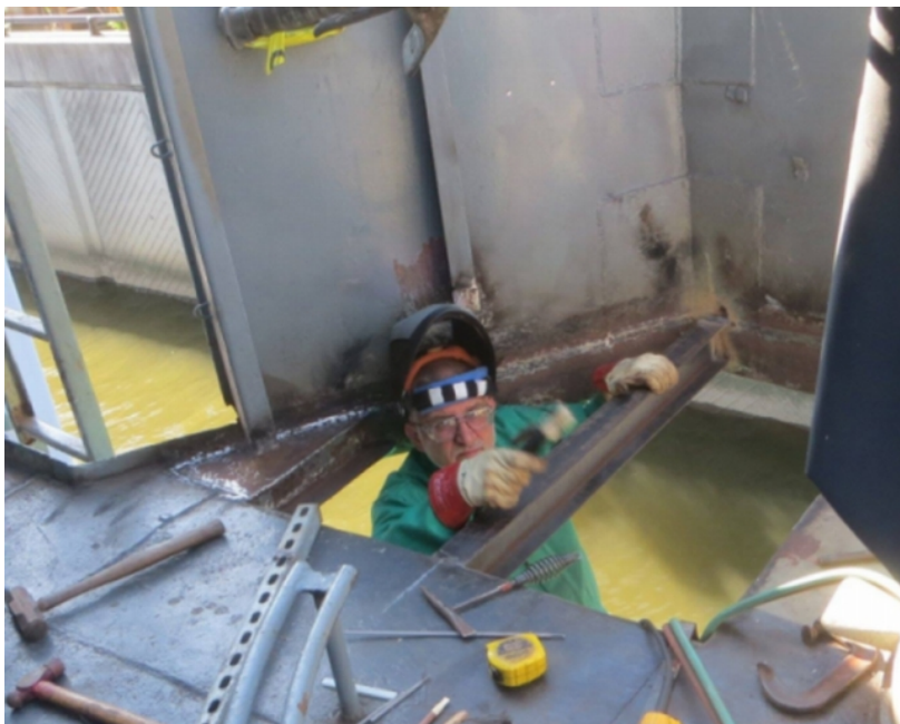
Tom Skufca and Laird Confer replaced a wasted section of deck.
