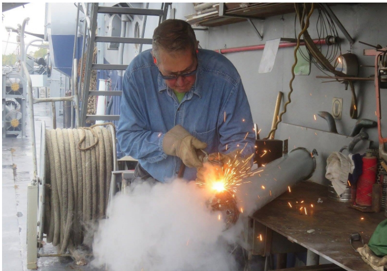
Danny Statile repairing a 20mm cooling tube.
