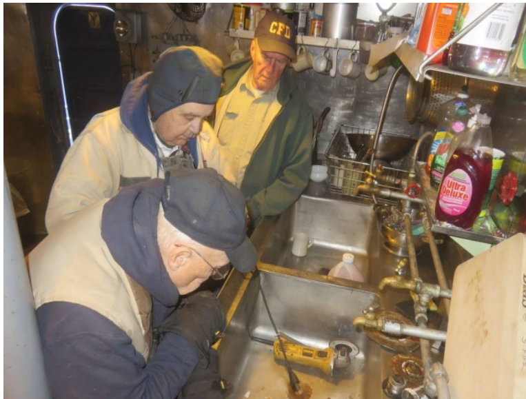
Planning the galley sink drain repair.
