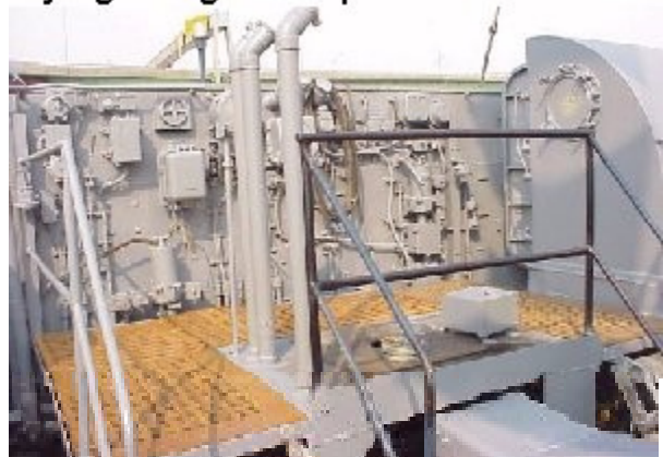
Flying Bridge after primer coat.
