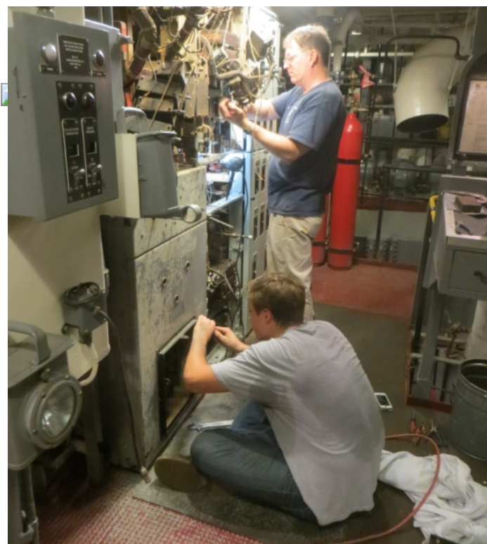
Progress on the emergency diesel distribution panel.
