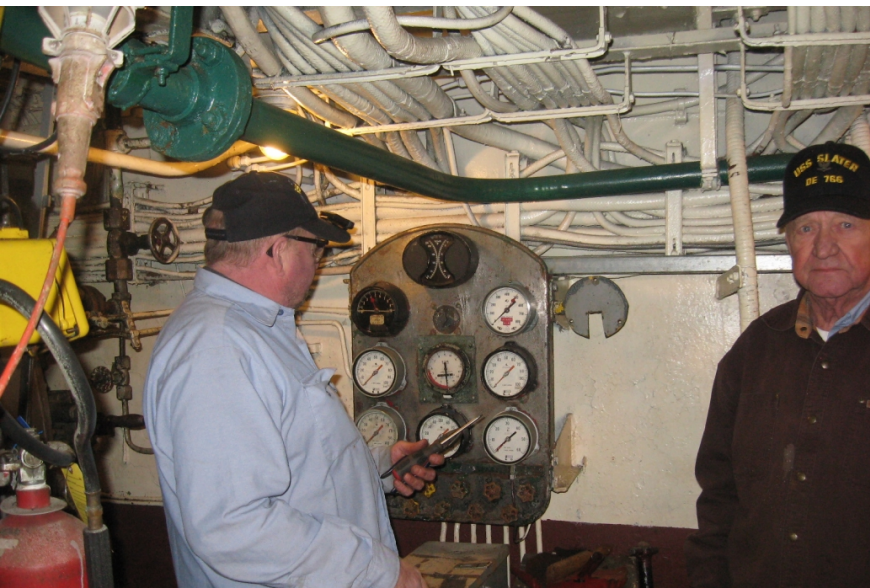
Engineers Mike Dingmon and Ken Myrick restoring the B-3 instrument panel.
