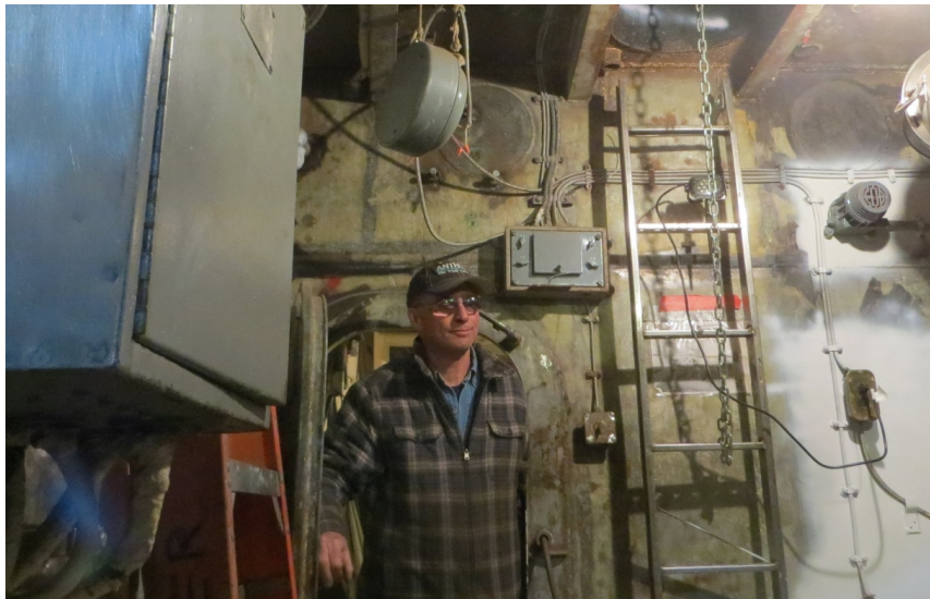
Gary Sheedy inspects the progress in the steering gear compartment.
