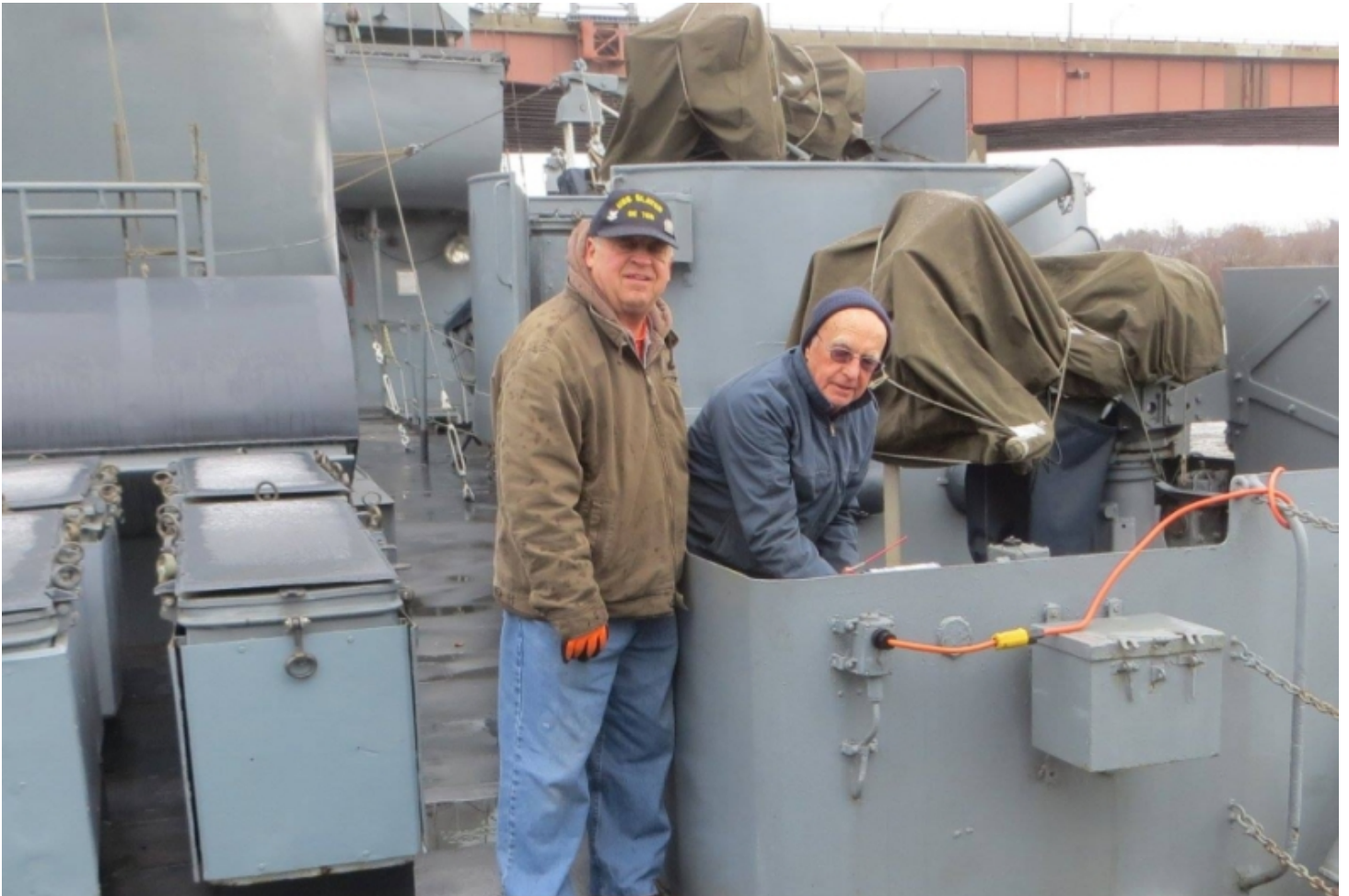
Walt Stuart and Larry Williams hooking up power for circulators that protect the hull from ice.
