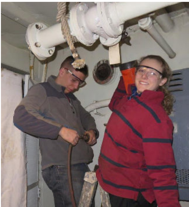
Work continues as RPI Midshipmen removed another section of firemain.
