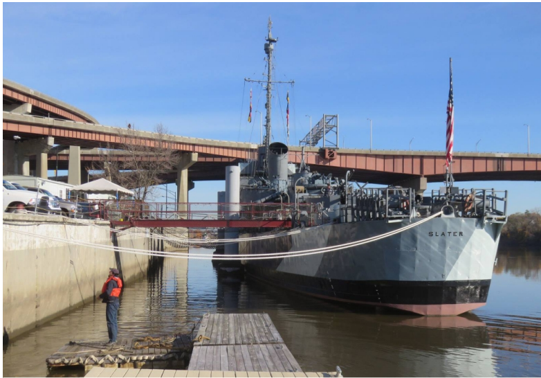
Stern view as the paint float is moved close to the sea wall.
