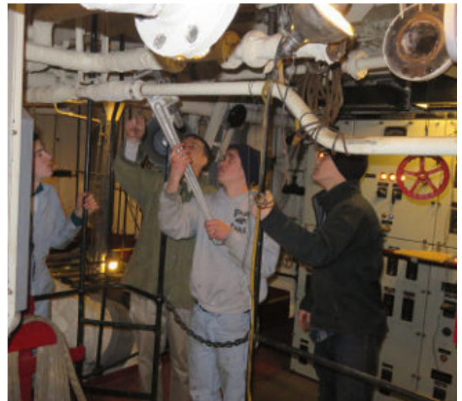
Barry Witte and his students continue their efforts to cool the emergency diesel generator off the firemain.
