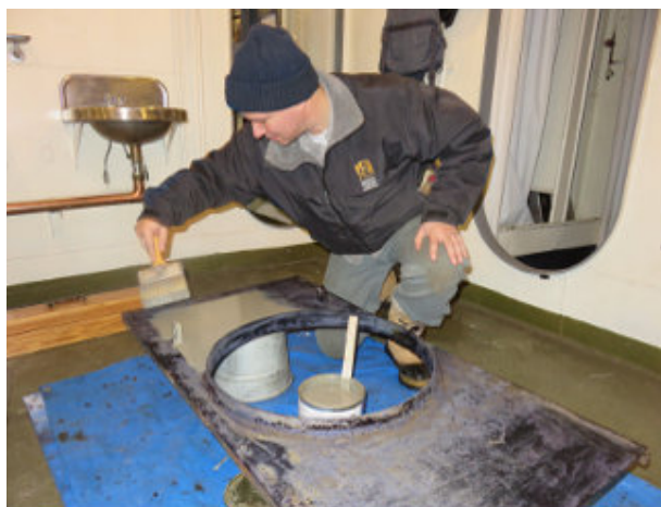
Paul Guarnieri priming the new scuttle for the gun three tub project.
