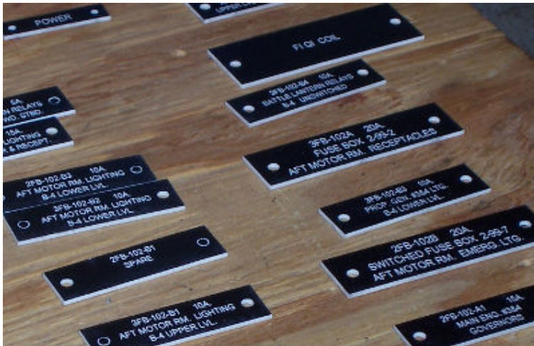
New tags for the electrical panels.
