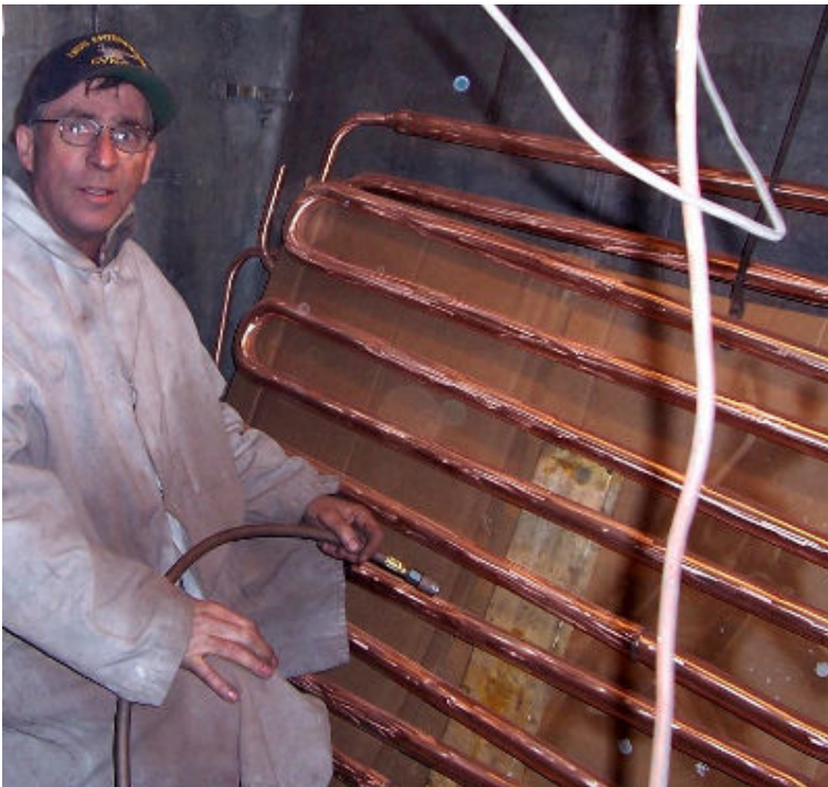
"I'd rather be on a cruise ship." Gary Sheedy polishing the reefer coils.
