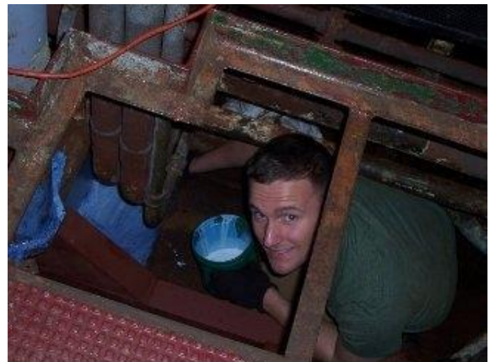
Applying the Corro Seal.
