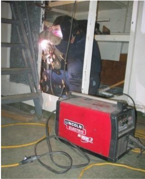
and "Super Dave" Mardon welding up the supports.
