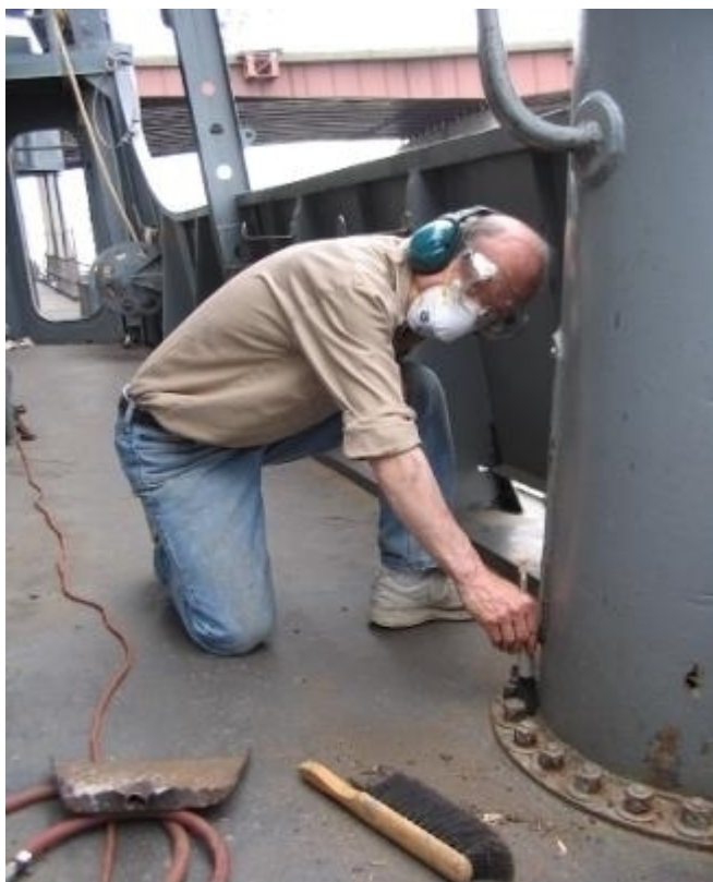
Gary Dieckman working on the davit base.
