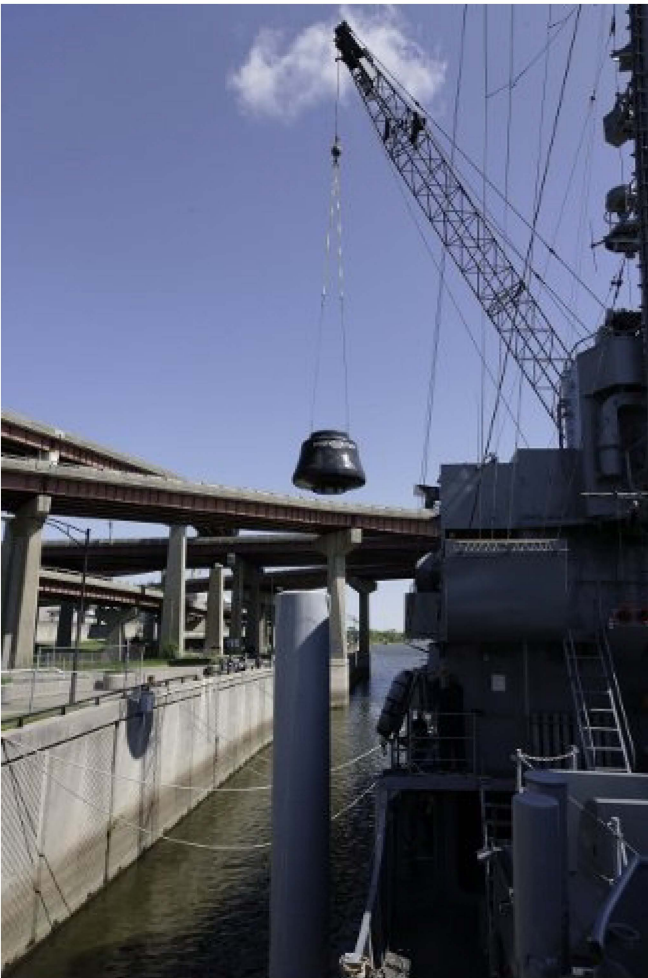
The final stage of building the mooring dolphins...
