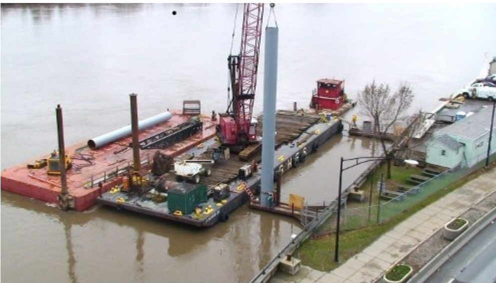
The mooring pilings under construction. Photo by Rich Aubin
