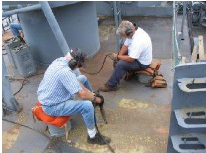
Chipping continues on the O1 level aft.
