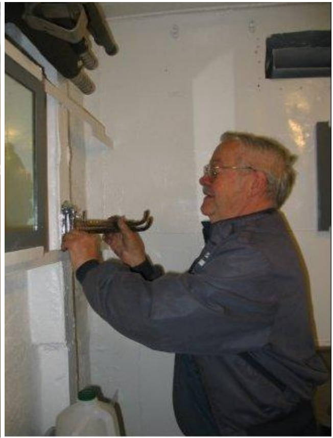
Karl Herchenroder installs refurbished towel racks in the crew washroom.
