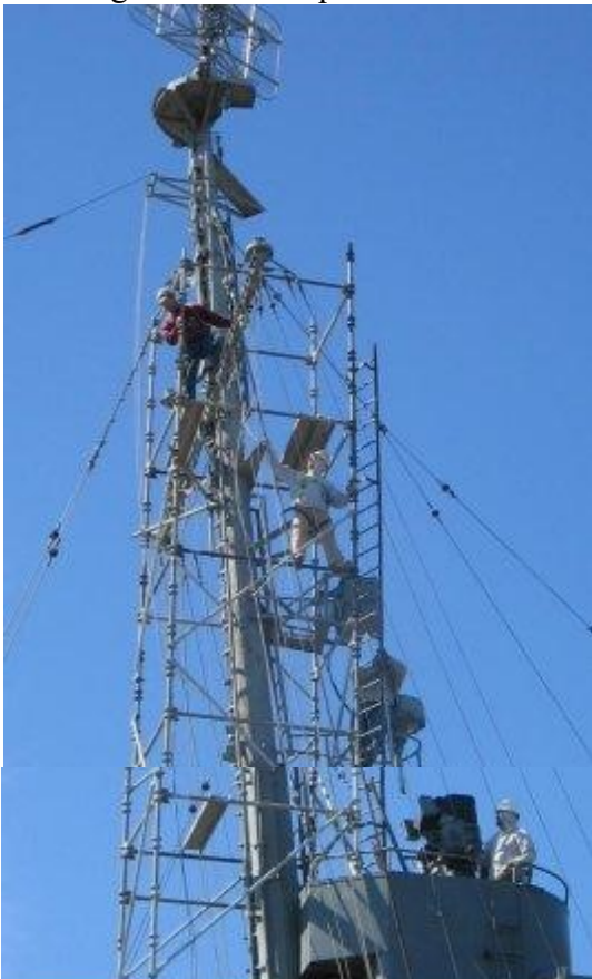
Getting the scaffolding up.
