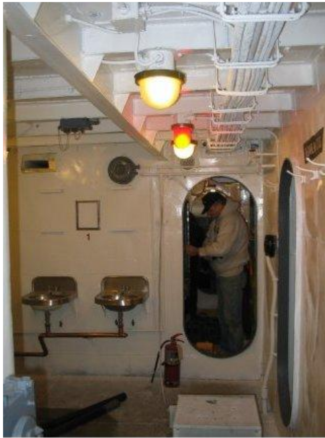
Gordon Lattey works on an electrical box in the aft passageway.
