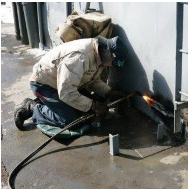
While Tim Benner cuts some wasted metal out of the aft head...
