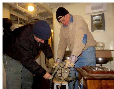
Paul Guarnieri and Bill Holt repairing circulators damaged by the ice.
