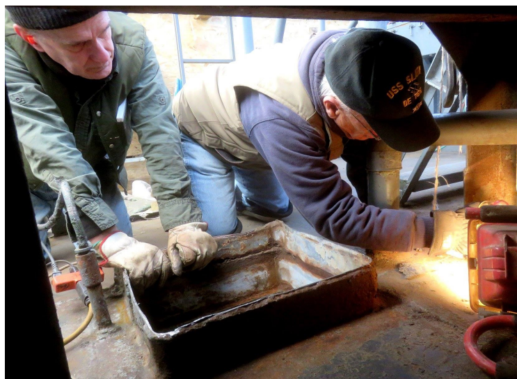
Chuck and Dave removing the CIC vent duct.
