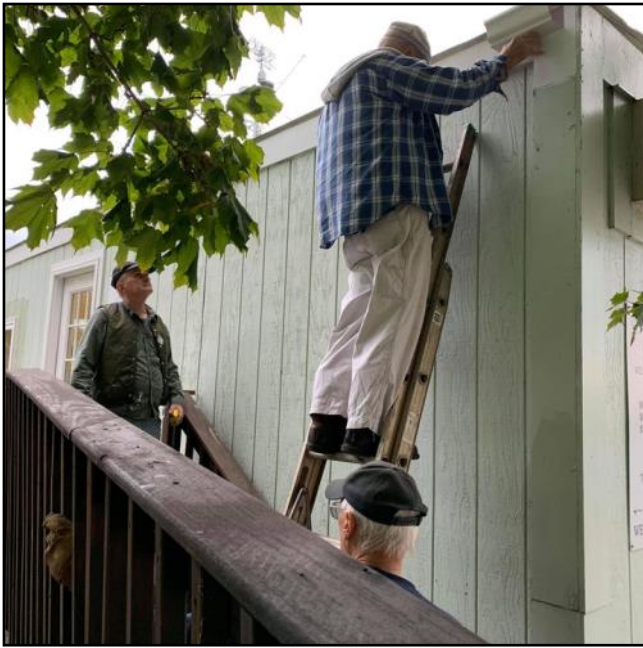
Chuck, Doug, and Dave working on the trailer.
