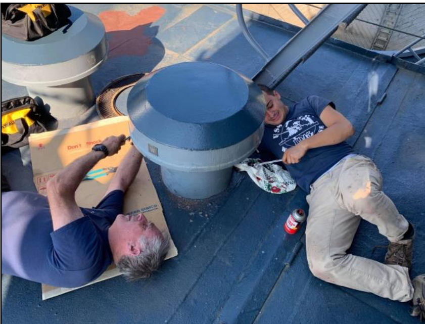
Gary and Thomas start disassembly of the forward galley supply vent.
