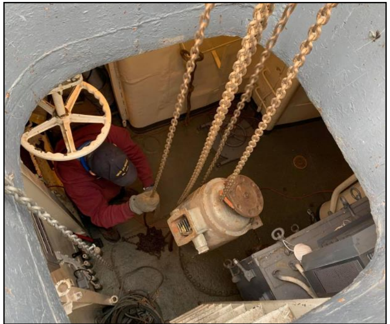
The first move of the motor generator set.
