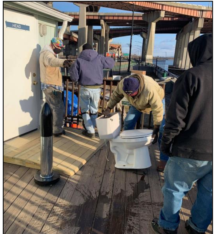
The crew made repairs to the commode in the shore head.
