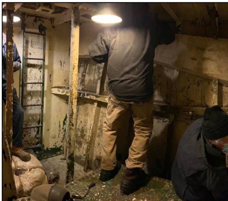
Ron, Tommy and Bill scaling in the Bosun's Storeroom.
