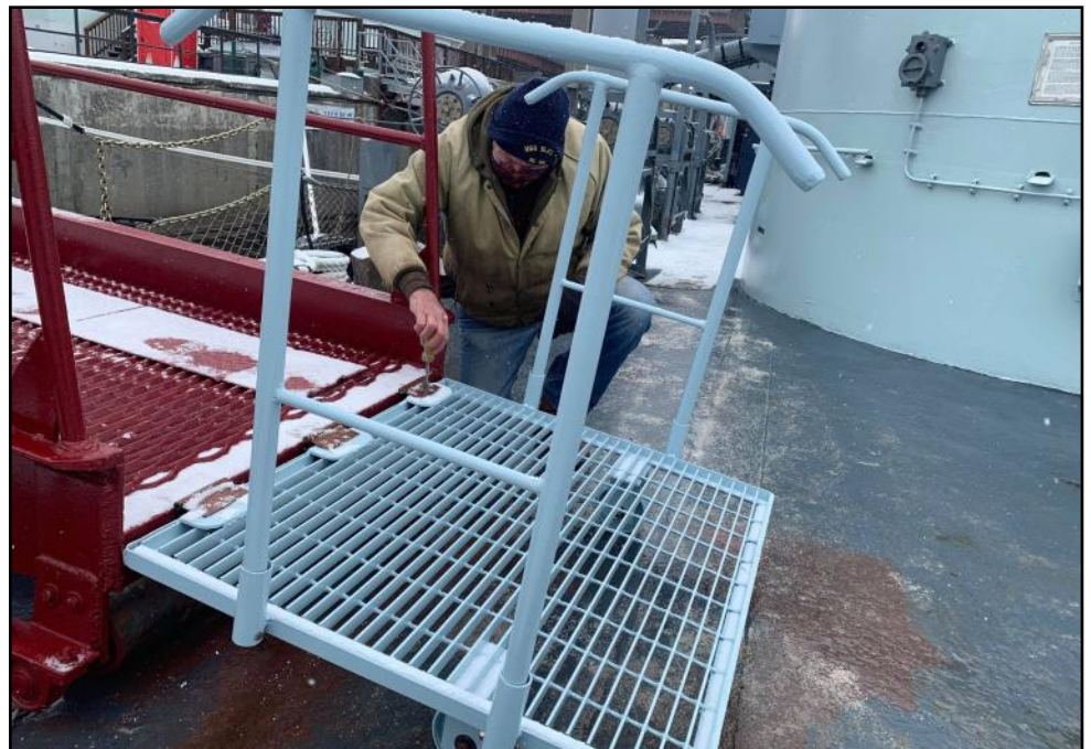
Danny finished the new ramp for the aft gangway project.
