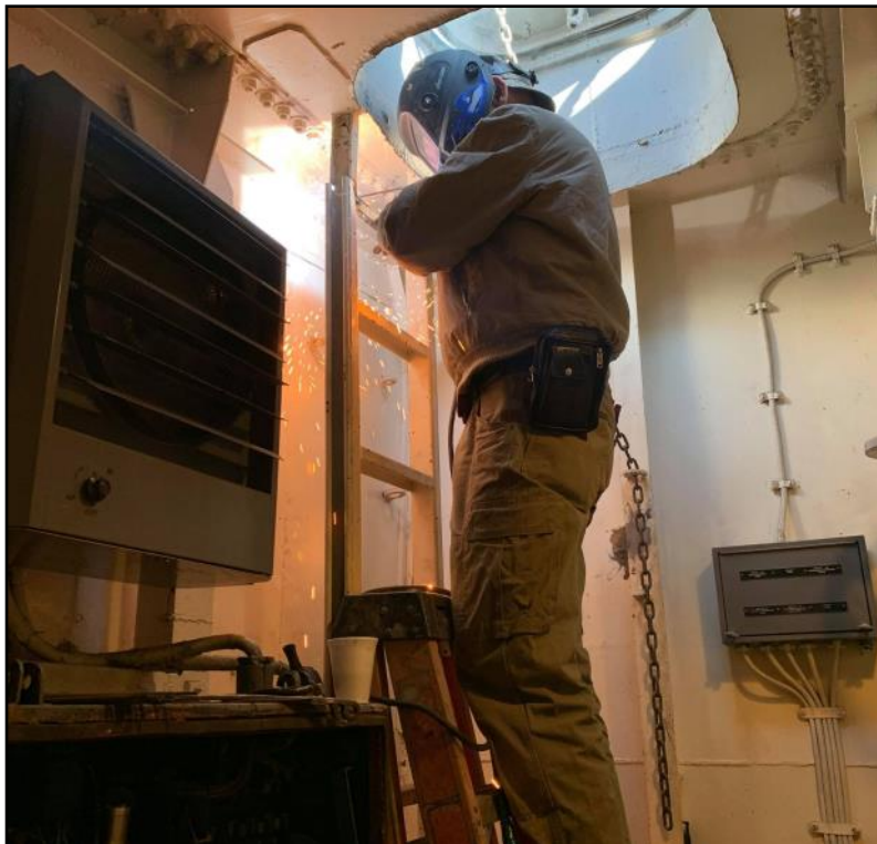
Tim Benner is welding the missing ladder rung.
