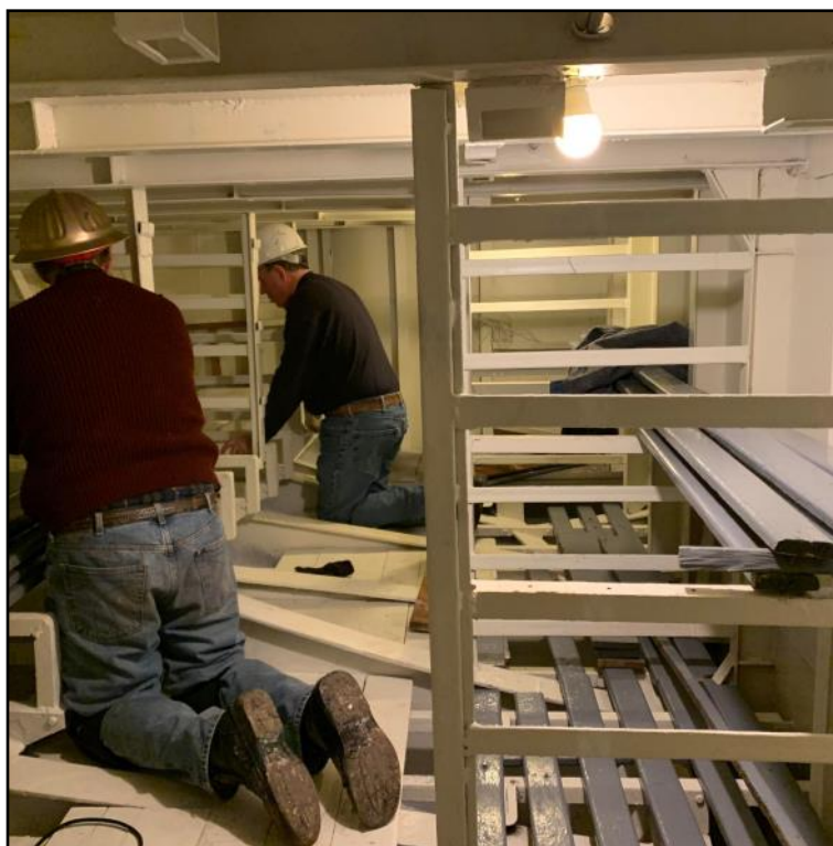
Ed and Dennis have just about completed the storeroom .
