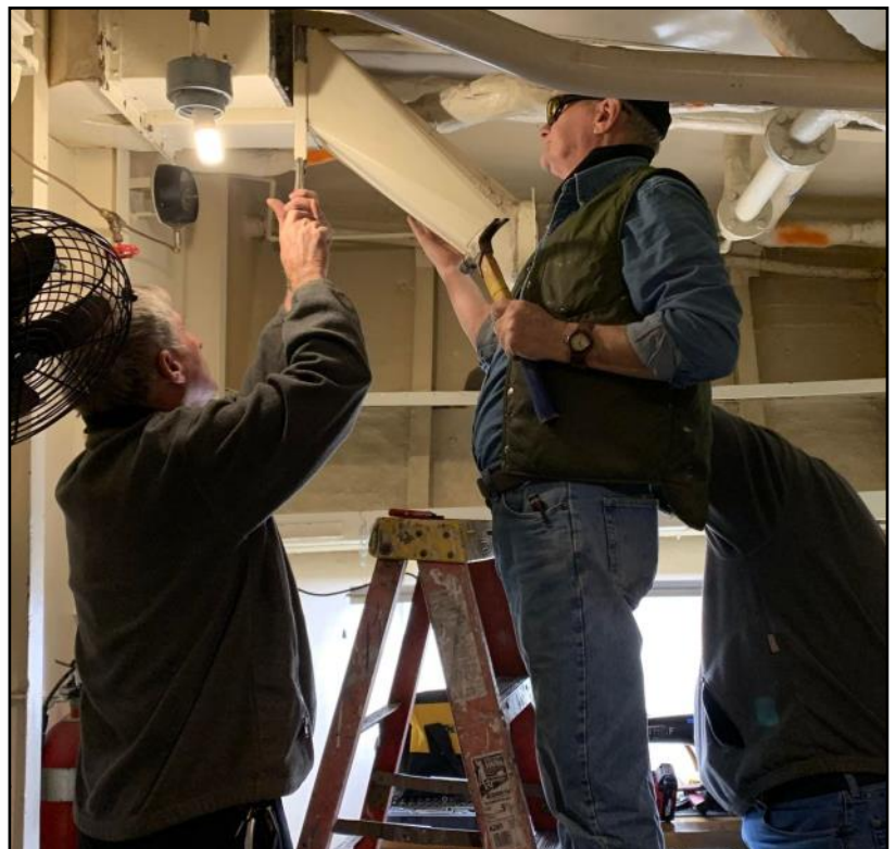
The shipfitters continued ductwork removal in the CPO passageway.
