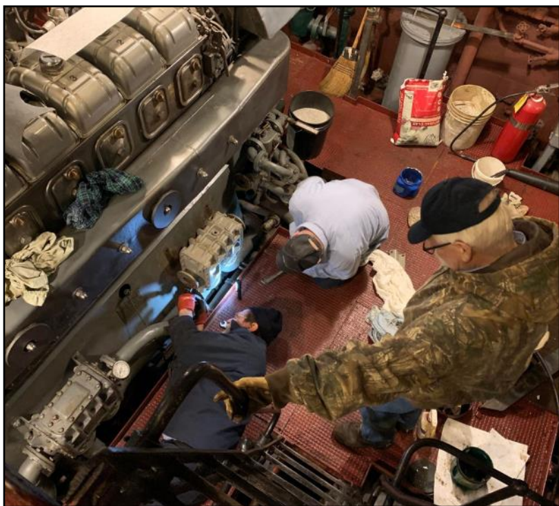
The Engineers continued the oil cooler change out.
