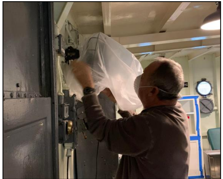
Walt masked the compartment fans in preparation for future spray painting.
