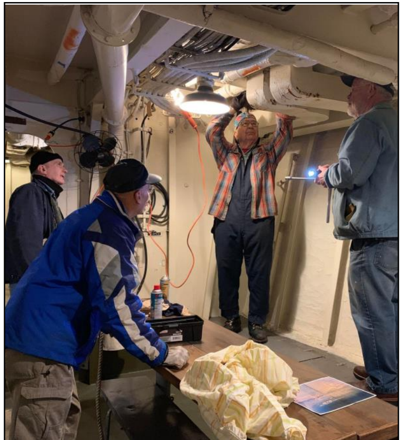
"This ductwork isn't original to the ship, so it's coming out."
