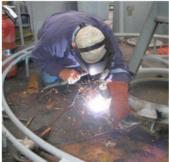
Clark Farnsworth welds up a hole in the deck. Did we mention he's 84!
