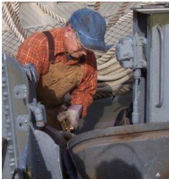
Laird Confer welding up a davit socket.
