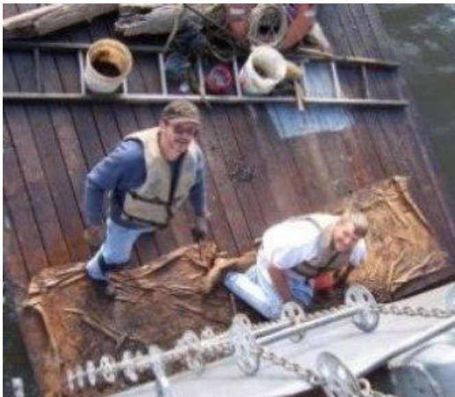
Ron Prest and John Yocum working the starboard boottop.
