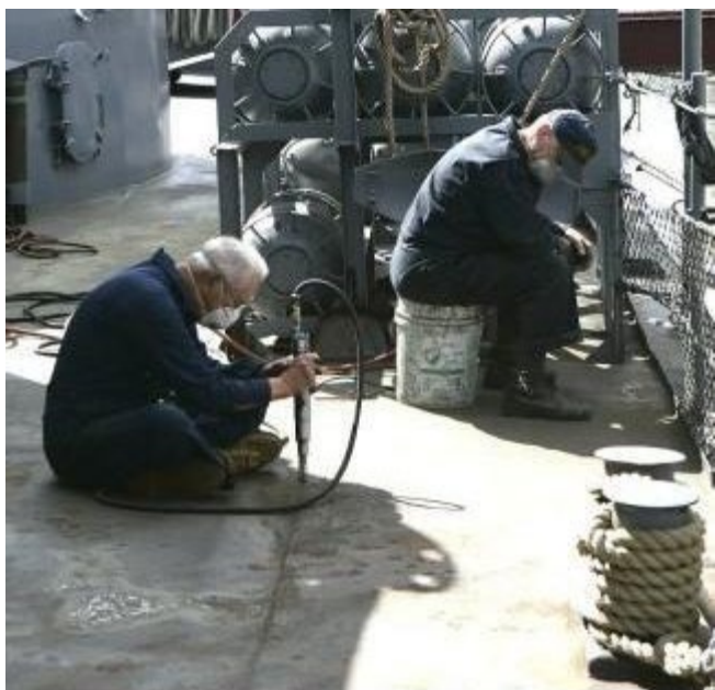
Guy Huse and Jim Ray chipping aft.
