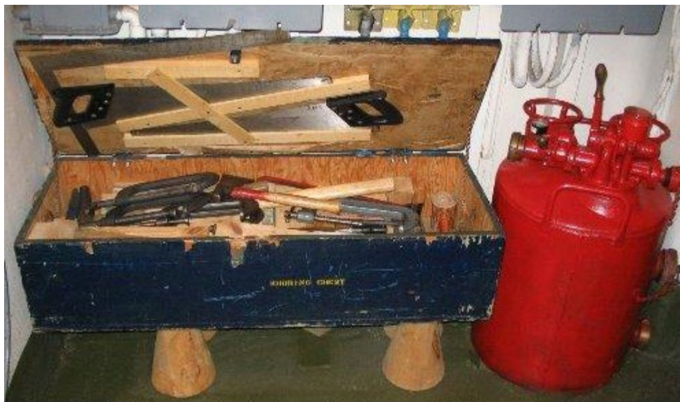
The restocked Shoring Chest sits next to the repainted Foam Generator.
