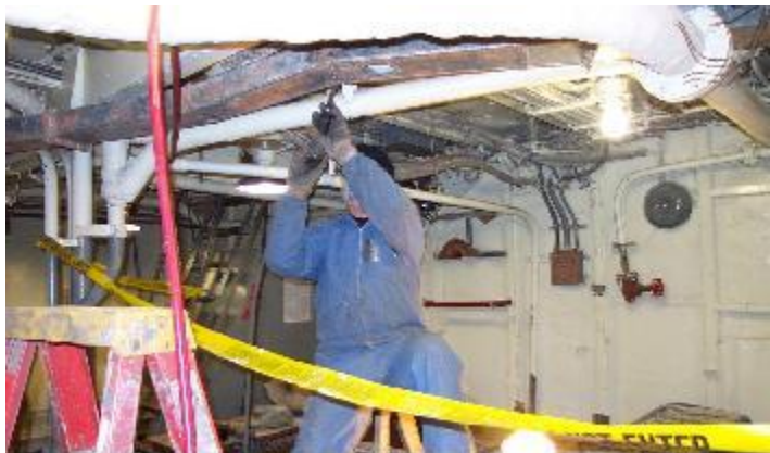
Chipping on the messdeck.
