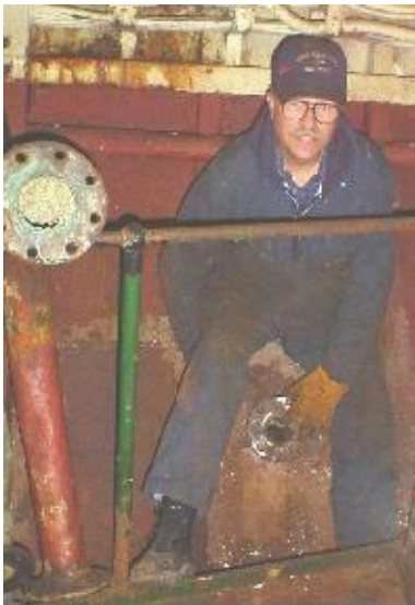
Larry Lachance replacing bolts on a sea suction.
