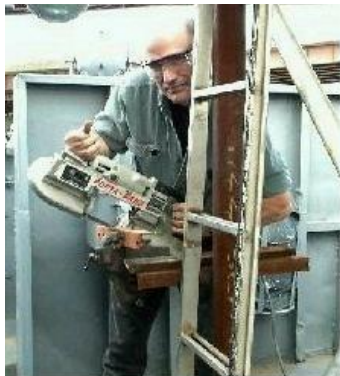
Chuck Teal working on the platform.
