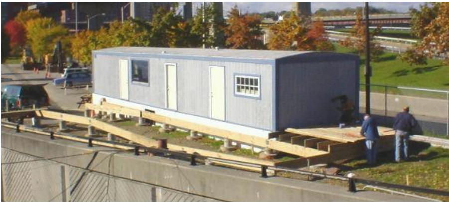
Progress on the trailer deck.
