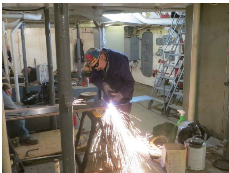
Doug Tanner cutting metal for the bunk locker repair.
