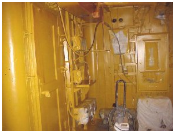
Prime Coat in Radio Central, Dec 99
