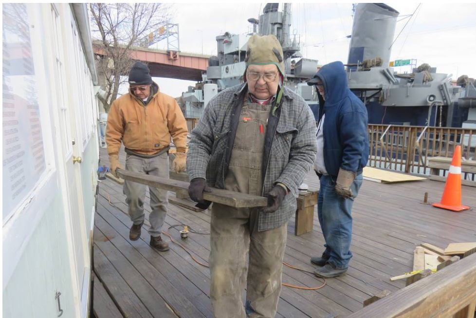
Doug Tanner and his crew replacing deck planks.
