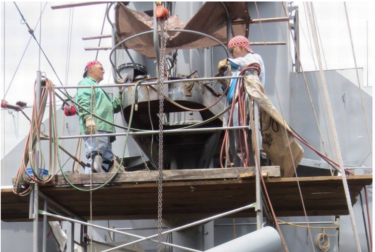
Progress continues on the RDT platform.
