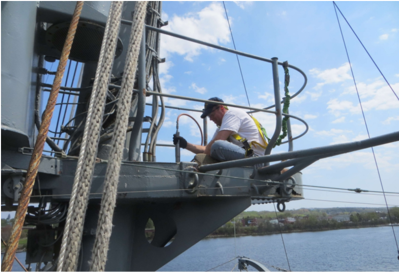
Scott McFadden working on chipping paint.
