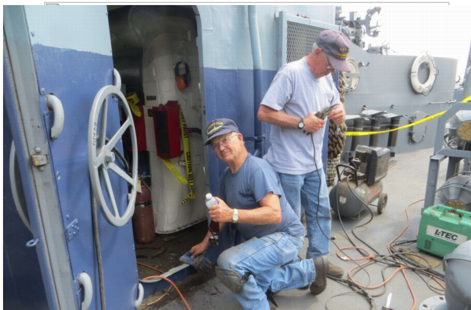
Laird Confer welding outside the aft passageway.
