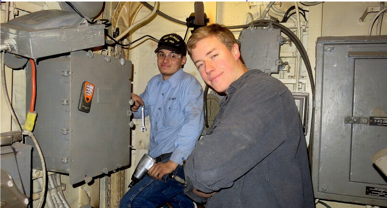
Thomas Scian and Jim Lenden working on the aft expansion joint.
