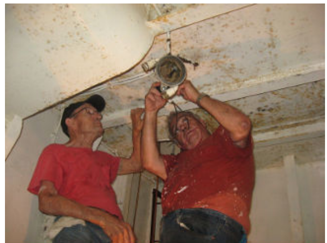
Ernie and Anthony replacing a light fixture.
