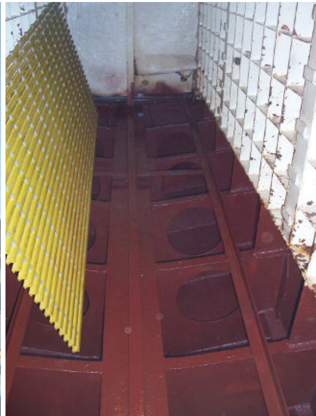
The depth charge magazine bilge after scaling and painting.
