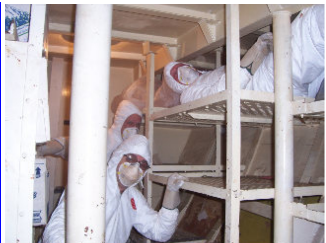
The insulation gang.
