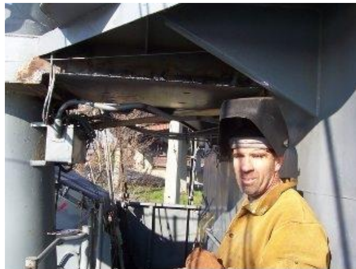
Joe Delberta works on repairs on the signal bridge.
